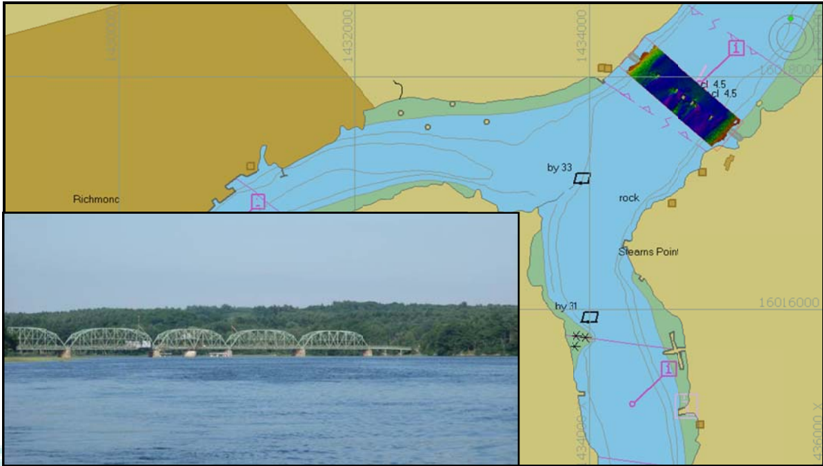
Figure 2. The location of the recent survey of the Richmond Bridge is shown on NOAA Nautical Chart US5ME18M. The inset photo is an image of the Bridge looking upriver from the town of Richmond.
