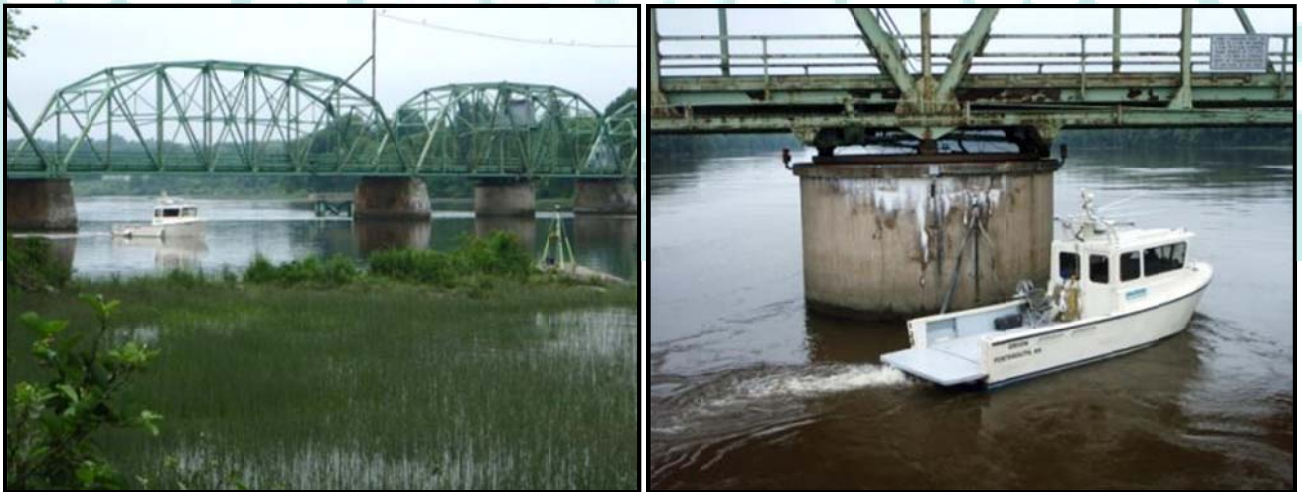
Figure 3. In the left photo, Orion is maneuvering near the eastern side of the Richmond Bridge during survey operations in July 2010. The RTK DGPS base station can be seen in the foreground set-up on a survey monument that was established by ME DOT. In the right hand photo, Orion is maneuvering close to the center turnstile support during survey operations.
