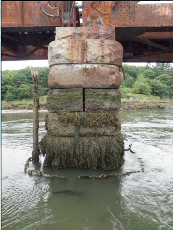
Figure 7. The top photo shows the center support for the Sheepscoot River Railroad Bridge while the photo at left shows a close-up view looking upriver at the support. The two point cloud data images include an overhead view and a rotated view looking downstream. Some Initial concerns about the wavy appearance of the point cloud images were resolved at low tide when the deteriorating remnants of the original sheet pile form could be seen at the water line. The point cloud results reflected the sheet pile form and not the main stone supports.
